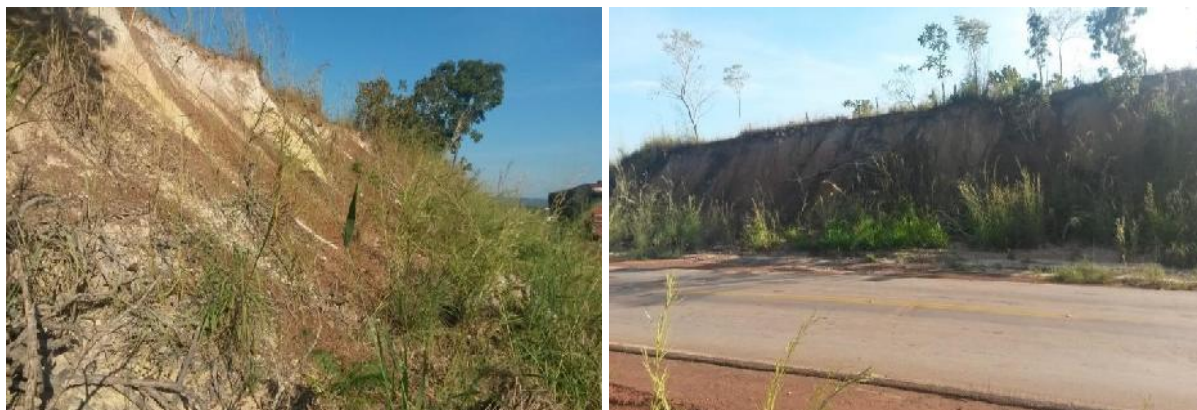
Foto 101 e 102: Km 15,8 a km 15,54 - C=100,0 m, H= 4,0, e L= 1,0 m
